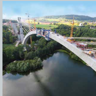
— The viaduct over Froschgrundsee: 798 m long, 65 m high, concrete arch with 270 m spans.
